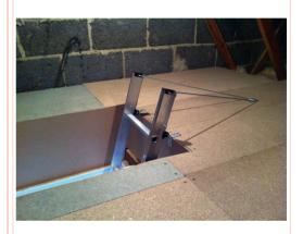
(3) You can fix a ladder on to a joist and stow it away from the deck.
