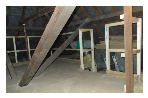
LoftZone has developed a raised decking for lofts, which protects insulation from compression, whilst allowing safe access to workers. Recent research by the National Physical Laboratory and Carbon Trust has shown that loft insulation is compressed in most UK houses, and that this reduces its effectiveness by 50-60%. The LoftZone raised decking won Best New Invention 2013 at the Ideal Home Show in London.
